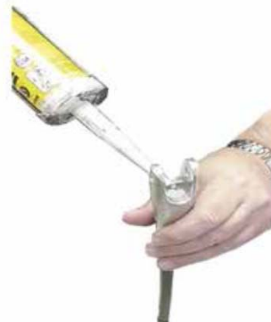
MOUNTING OF TERMINALS IN THE SYNTHETIC ROPE
